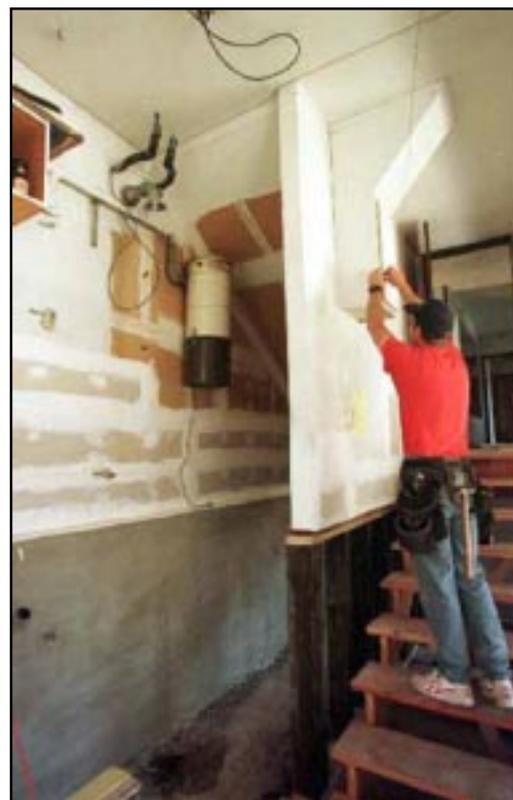
*Mitigate while rebuilding. Moving a water heater above ground level will help save the appliance and keep it working during a flood. FEMA News Photo by Gave Gatley.*
